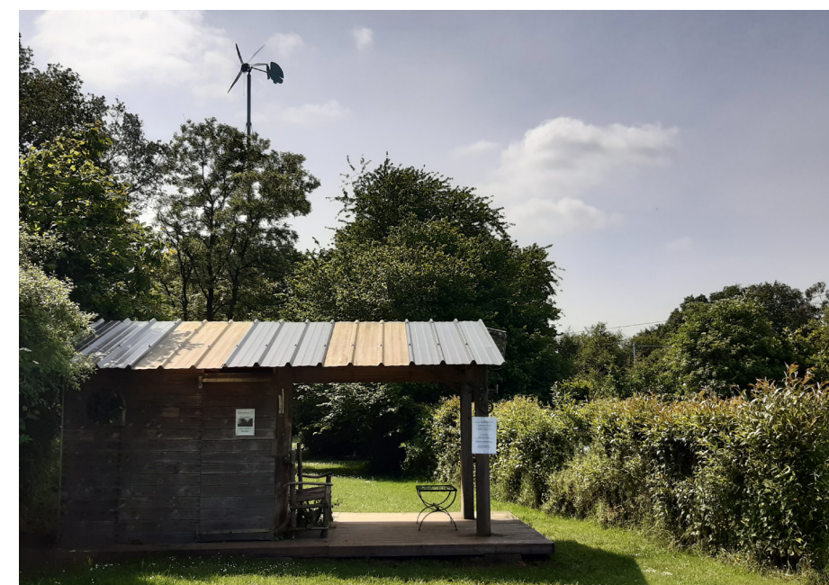
Dry toilets, solar showers, depurative hedge
